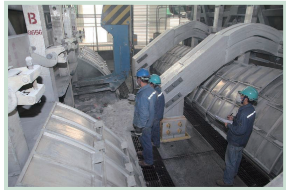
Electrolysis cell maintenance technique training
